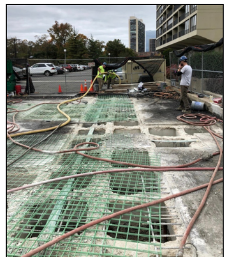
Rotting concrete had to be removed and replaced on the parking deck between Buildings 5 and 6. (Photo courtesy Al Fuentes)
